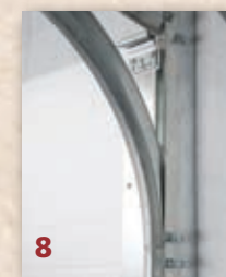
8 Continuous angle completely encloses the frame
